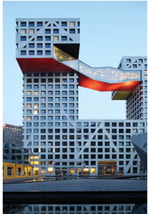
Above: Exterior views of skybridge connections Left Photo © Iwan Baan, Right Photo © Shu He Opposite Top: Building sections Opposite Bottom: Aerial view within urban context Photo © Shu He
