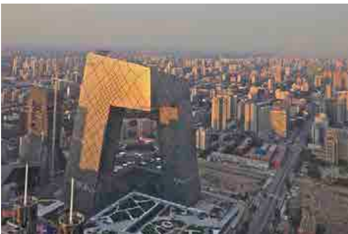
Figure 2. CCTV Headquarters, completed 2012. Source: (c) OMA Photography by Philippe Ruault.
