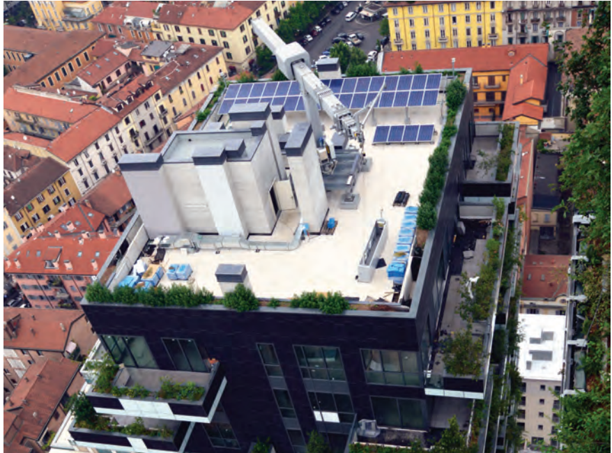
Figure 5.1 The telescopic arm on top of the tower that controls the basket lift for maintenance of the vegetation
