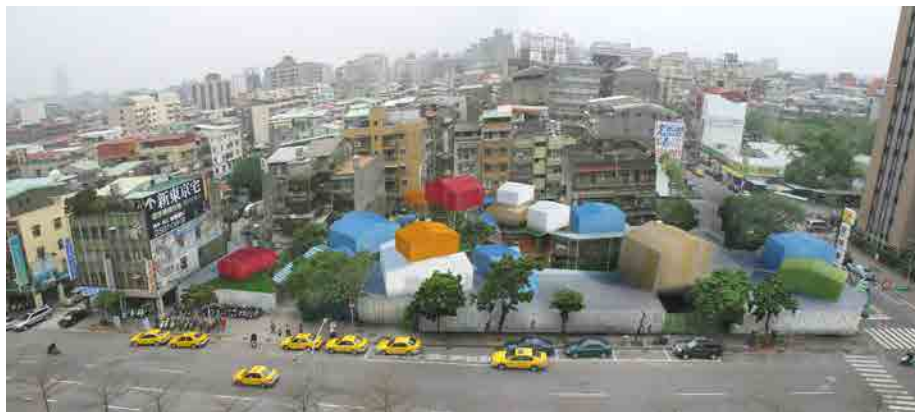
Figure 2. Additions on top of existing buildings in Taipei showing MVRDV intervention (Source: MVRDV) 图2. MVRDV设计后的台北现有建筑物顶部添加物 (来源: MVRDV建筑事务所)
