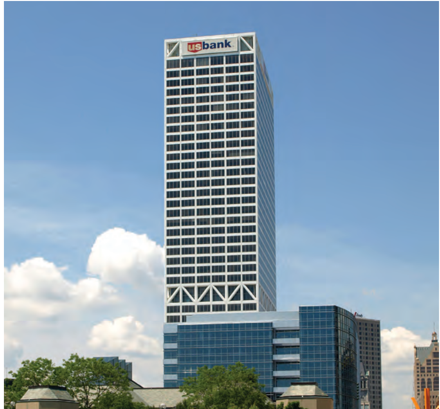
▲ Figure 4.2: U.S. Bank Center, Wisconsin. © Marshall Gerometta/CTBUH
