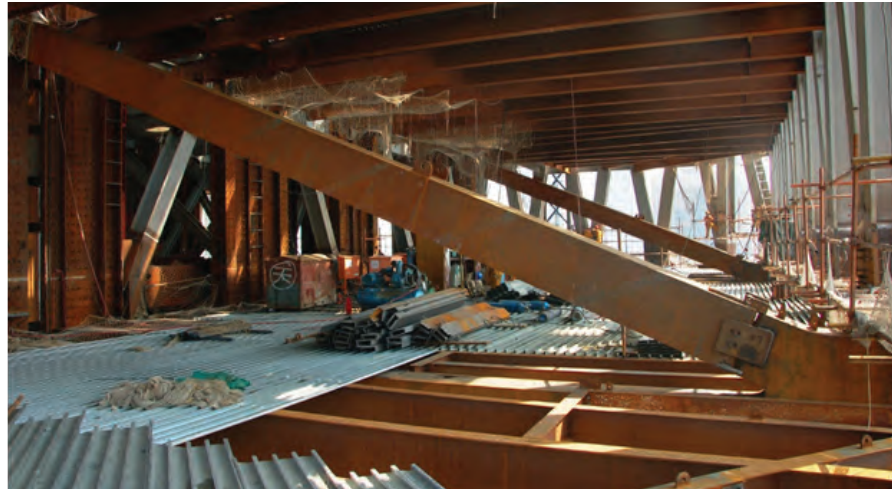
▲ Figure 3.2: Flexible outrigger used in China World Tower. [ed: © Arup]
