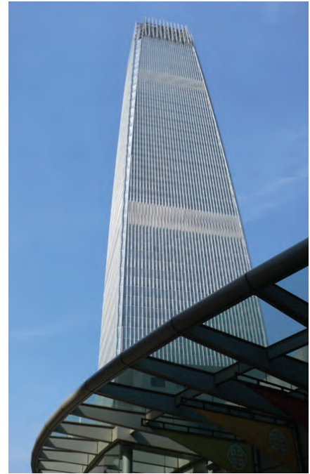
▲ Figure 3.1: China World Tower. [ed: © Goman, Arup]
