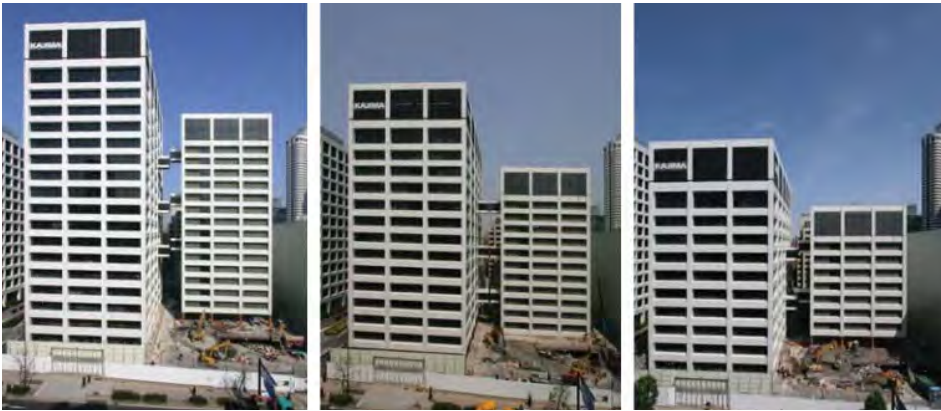
Figure 8.1: Kajima Demolition Method applied at the Kajima HQ, Japan Source: Kajima Corporation
