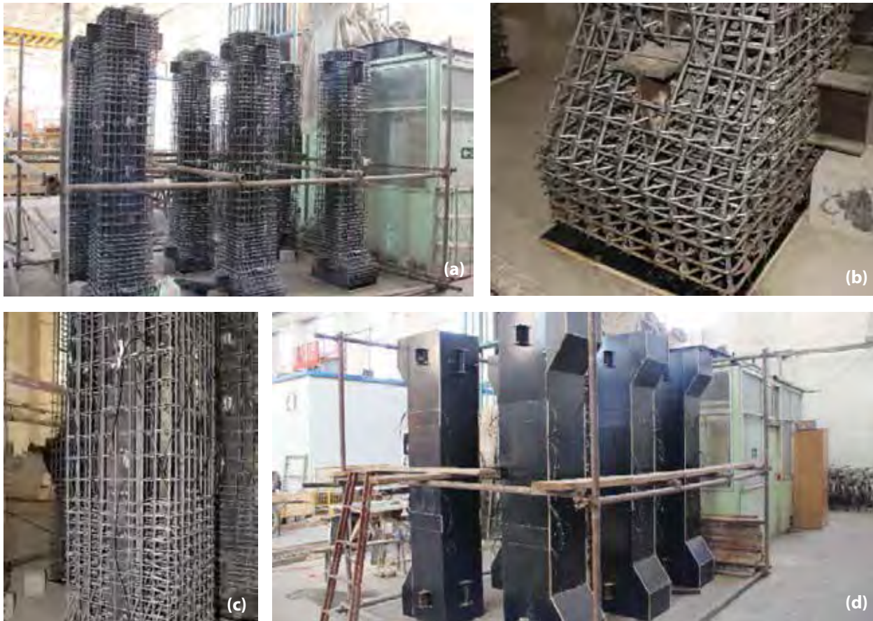
Figure 4. Specimen fabrication – static test, overview (a), bracket details (b), longitudinal bar details (c), and concrete mold (d). Source: CABR 2015
