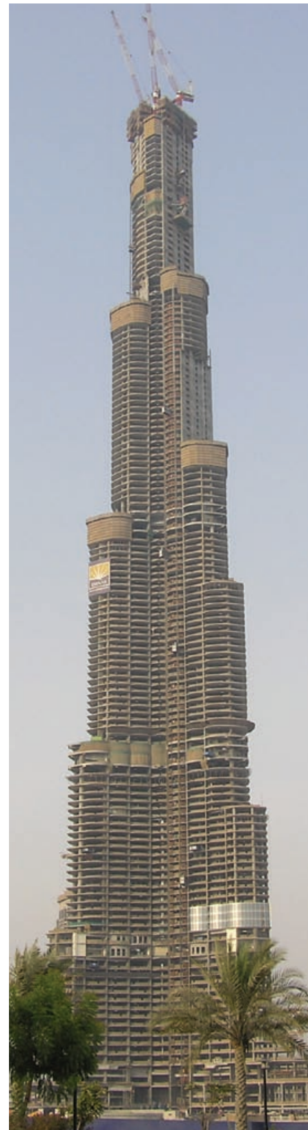
Fig 1. Burj Dubai under construction
