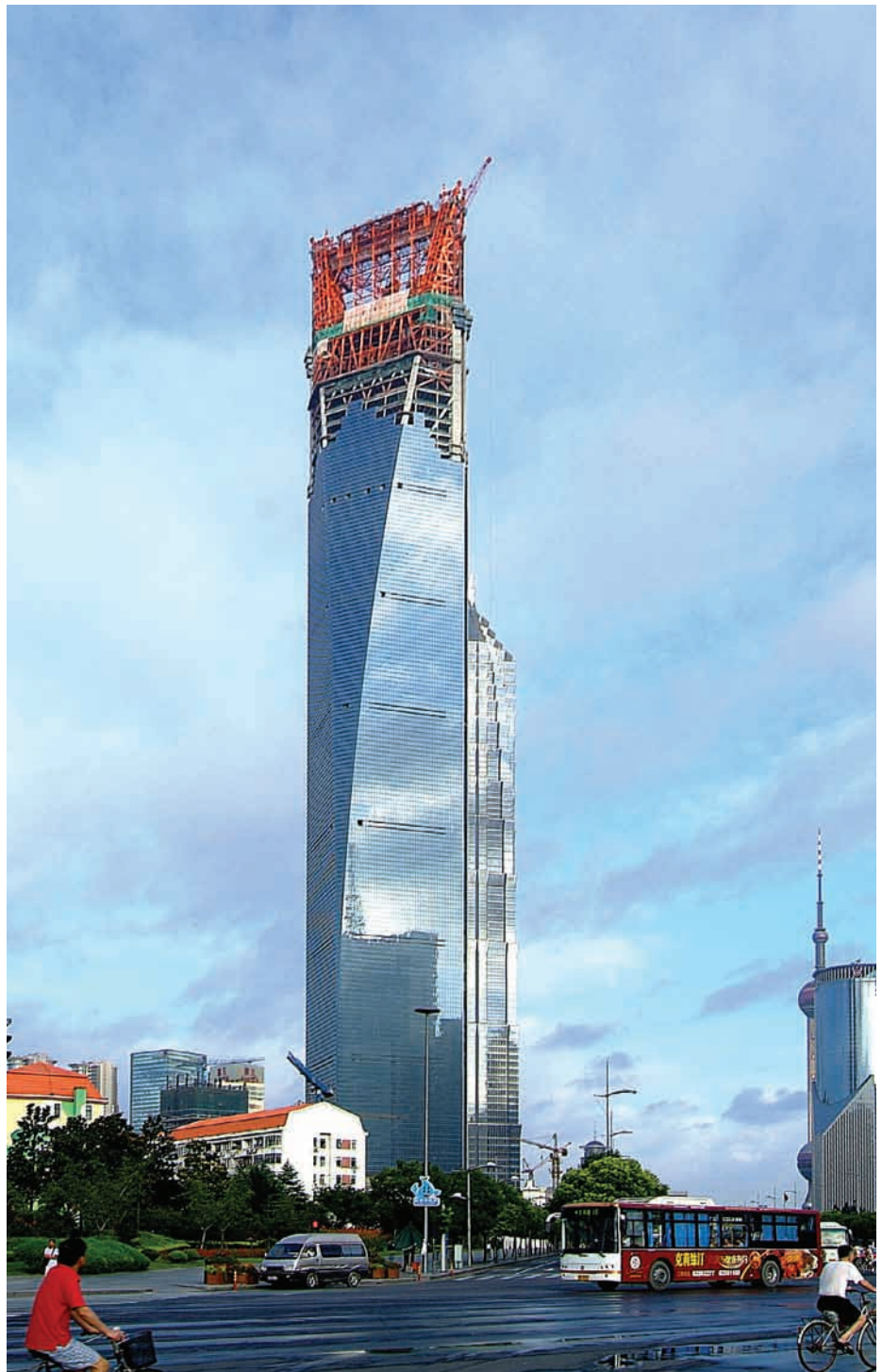
Figure 1. Shanghai World Financial Center nearing completion.
