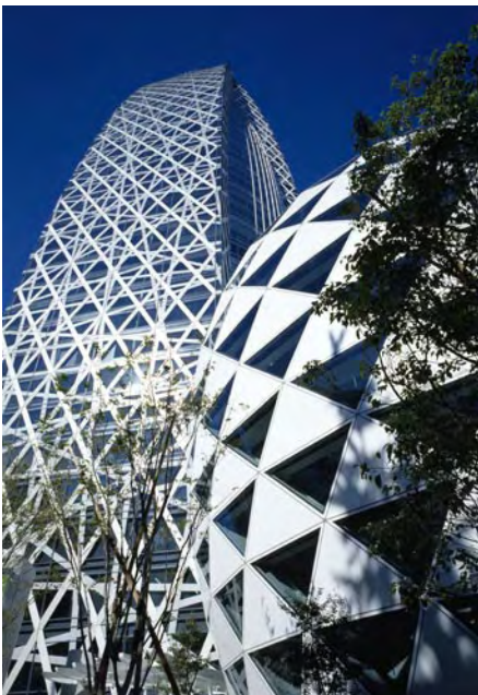
Figure 2. The low rise building adjacent to the high rise tower, houses two major auditoriums.
