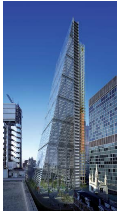
122 Leadenhall Street © British Land
