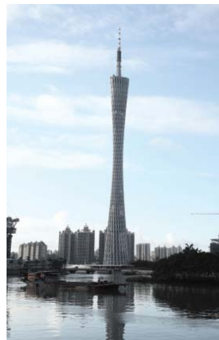
Canton Tower, Guangzhou, China © Information Based Architecture
