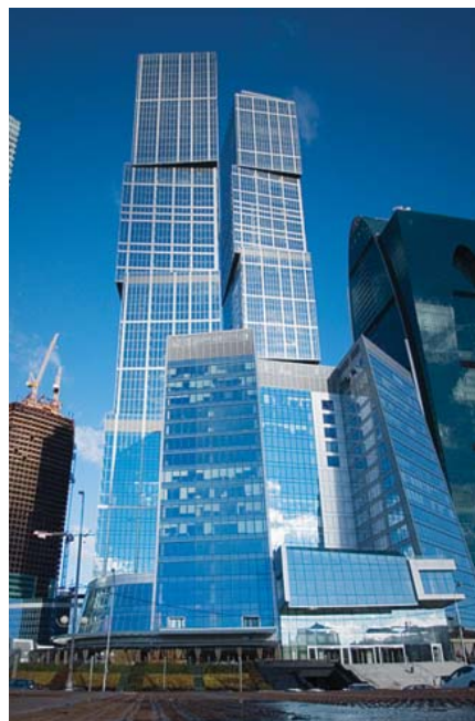
Figure 1. Capital City Towers © NBBJ
