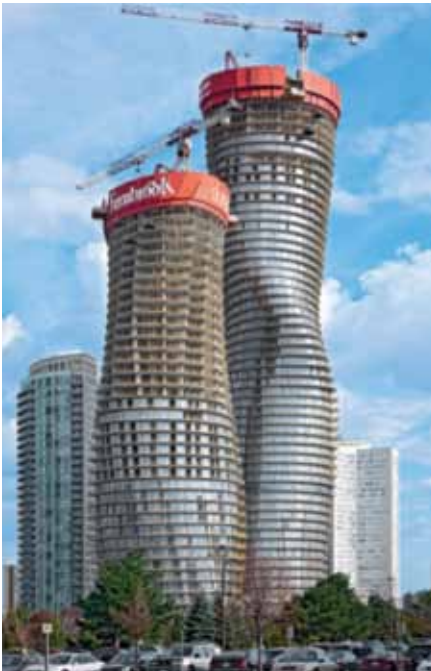
Figure 4. The towers' rotation difference. © PERI
