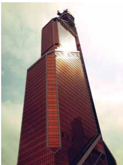
Mercury City Tower, Moscow. © Frank Williams & Partners
