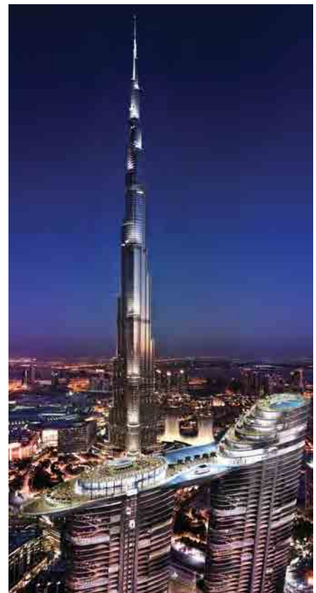
The Address Residence Sky View, Dubai. © Emaar Properties PJSC
