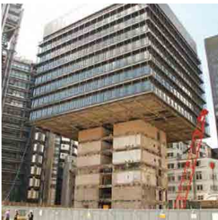
Figure 3. P & O headquarters being demolished from ground up. © BritishLand/Oxford Properties
