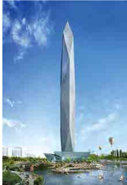
Cheongna City Tower Infinity, Seoul. © GDS Architects
