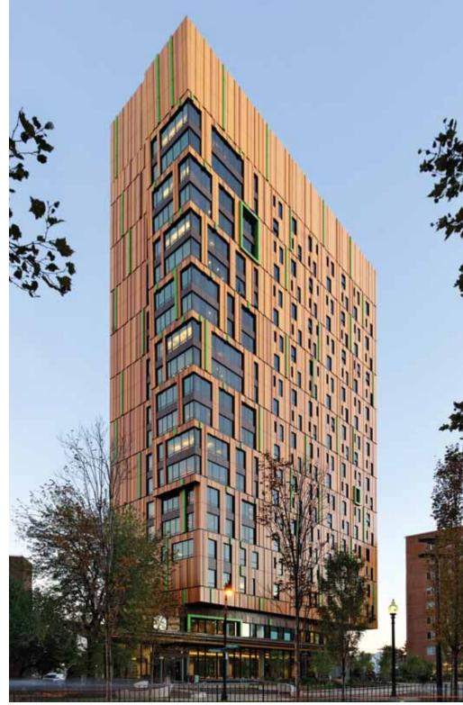
Figure 2. Windows configured in response to the passive daylighting techniques. © Chuck Choi
