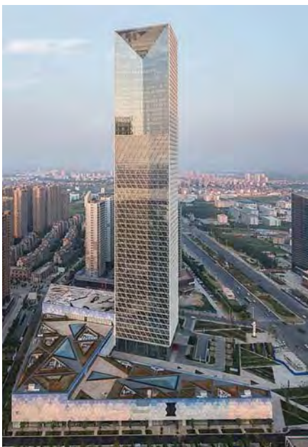
Jiangxi Greenland Zifeng Tower, Nanchang. © Lv Henzhong
