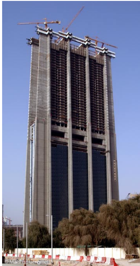
Tour 3: Index Tower under construction.
