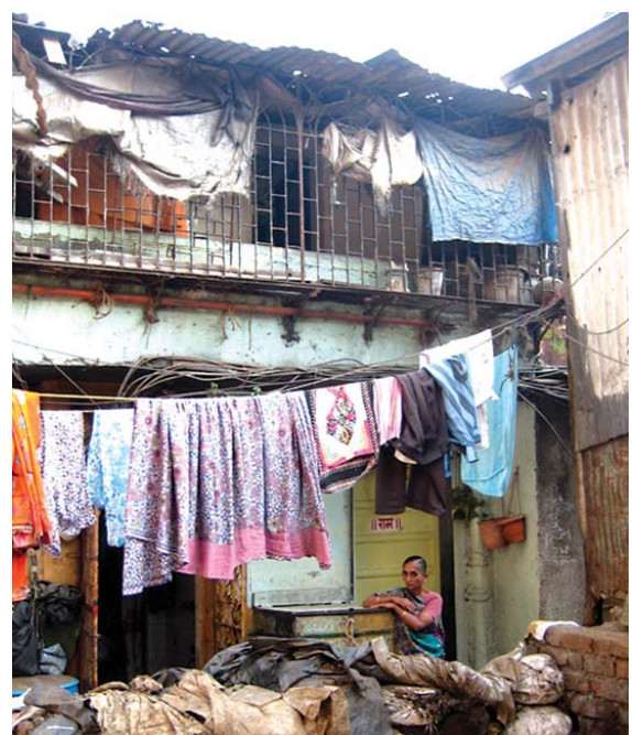
Hanging washed clothes on electrical cables.
