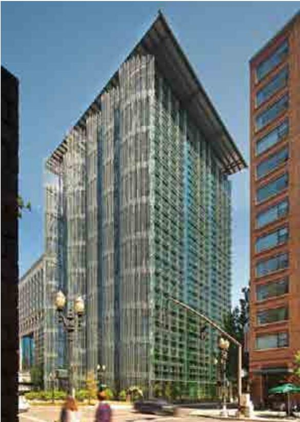
that the large fans for the previous forced-air cooling system could be removed. Additionally, removing the concrete façade panels simplified the seismic retrofit of the building due to the reduction of weight; the new façade system could be attached to the structural frame with a series of relatively short steel beams.
