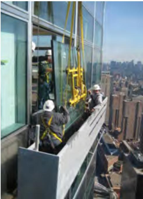
▲ Figure 3.1: Glass replacement is a common operation required of a façade access system. Courtesy of Lerch Bates, Inc.
