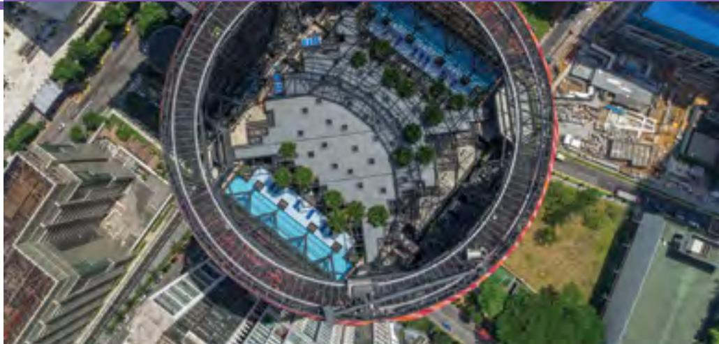
▲ Figure 3.1.1: A BMU is stored on the ring at the crown for when it is needed. © K. Kopter
