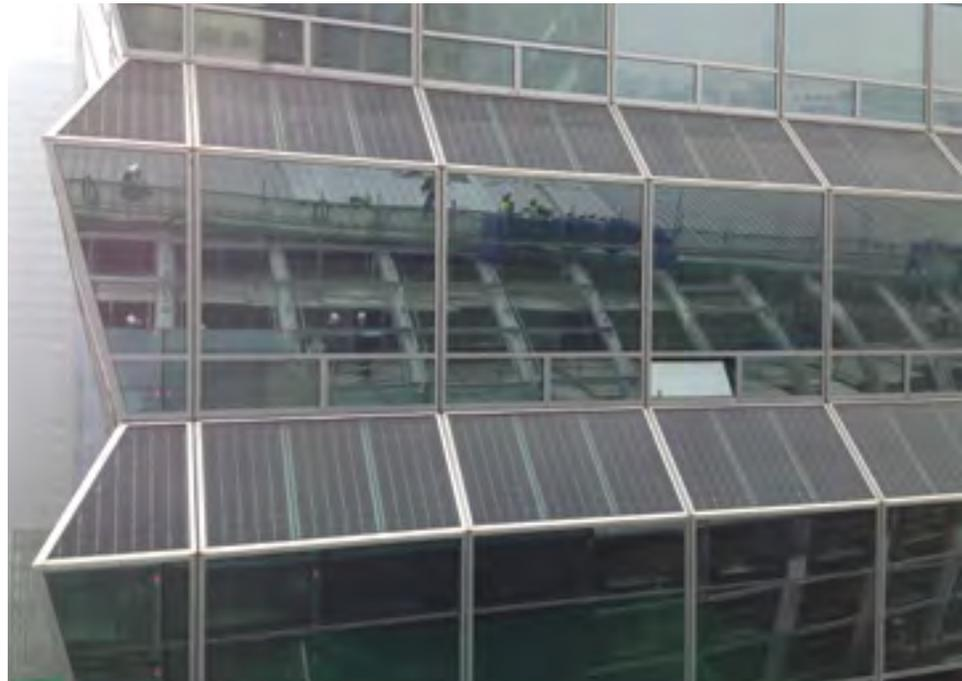
▲ Figure 3.2: Special building elements, such as PV paneling, must be considered in the initial BMS design analysis. © Adrian Smith + Gordon Gill
