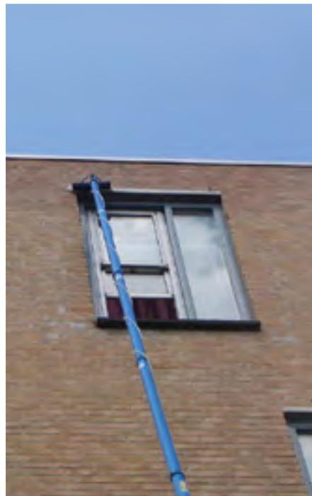
▲ Figure 1.1: Tucker Poles use a telescoping water line and brush to safely clean façades from several floors below.
