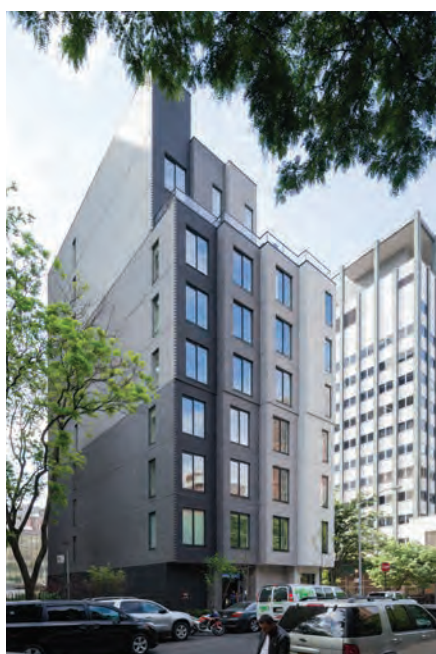
Figure 3. Street view of completed Carmel Place project. © Iwan Baan
