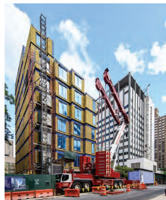
Figure 4. Modular assembly underway at Carmel Place.
