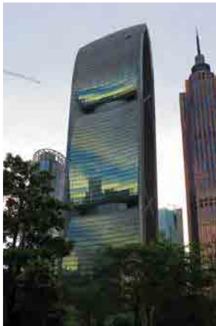
Figure 4. Pearl River Tower, Guangzhou uses its sculpted form to direct wind toward turbines situated at the recesses in the façade. © Tansri Muliani
