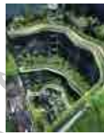
PARKROYAL on Pickering Singapore, 2012 Building Height: 89 meters Stories: 15
