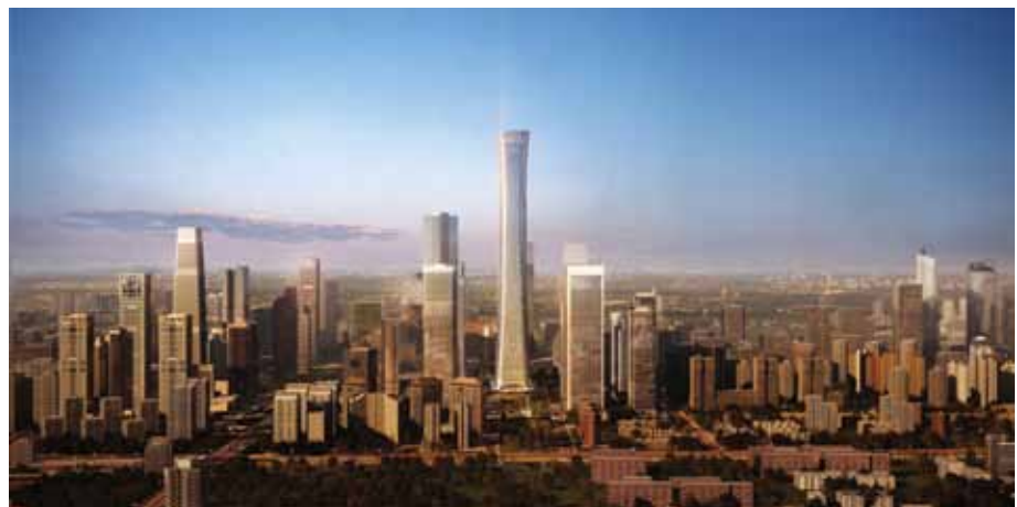
Figure 1. China Zun Tower, located in Beijing CBD. © KPF
