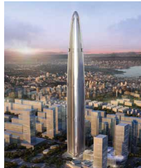
Figure 5. Wuhan Greenland Center's distinctive floor slots help to reduce the vortex shedding. © AS + GG Architects
