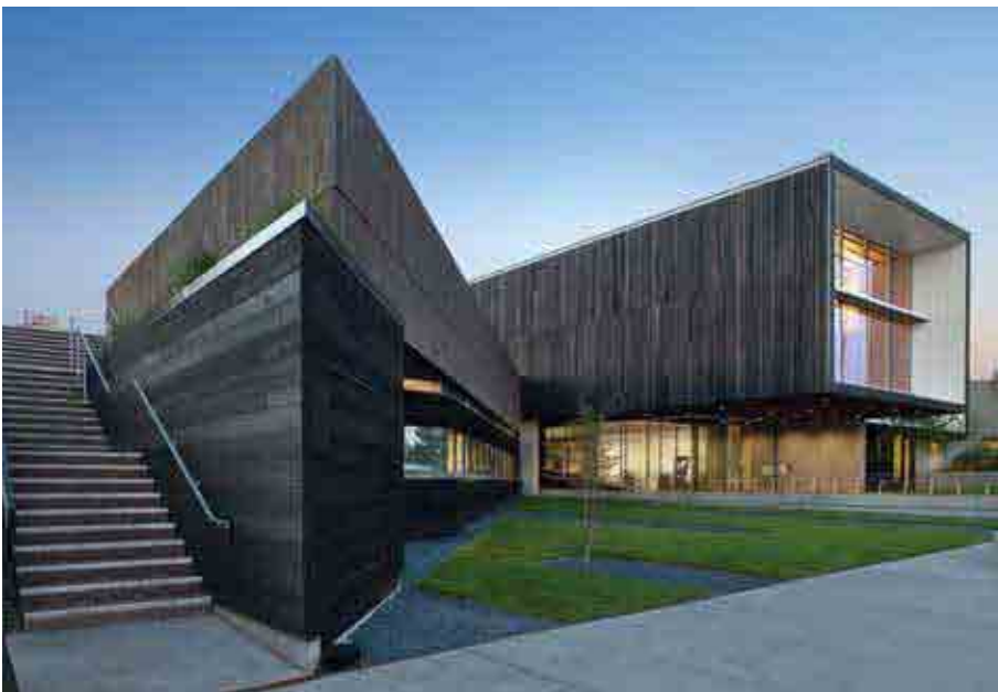
Figure 1. North Vancouver City Hall, Canada. © Michael Green Architecture
