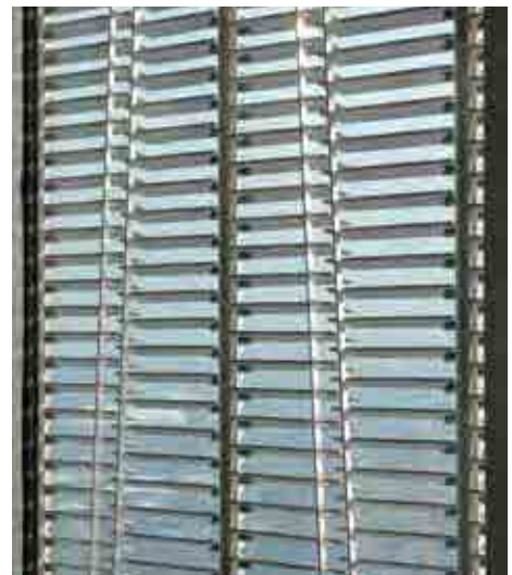
Figure 1. Type 316 stainless steel exterior sunscreens in varying styles were used on the ThyssenKrupp corporate campus to actively adjust to seasonal and weather conditions to reduce energy requirements. © ThyssenKrupp AG
