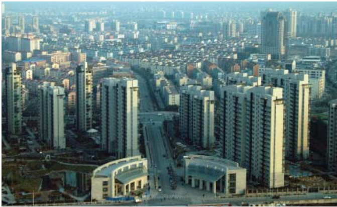
Figure 2. High-rise development in Shanghai. Note the relentless repetition of the freestanding towers and their angled relationship to the central avenue © Brian McMorro
