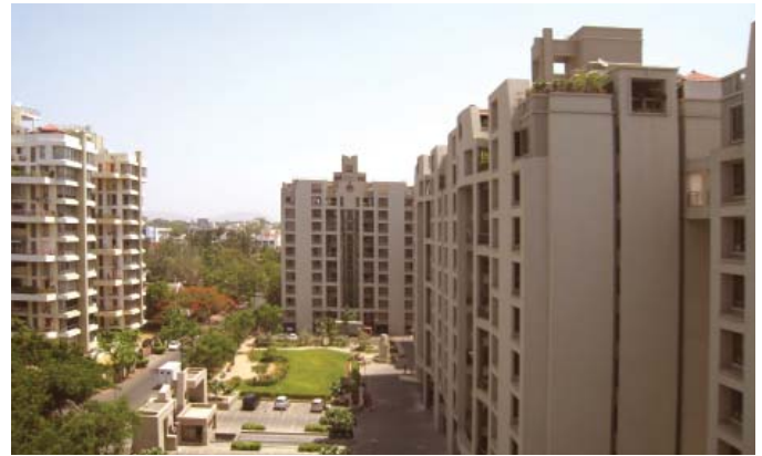
Figure 3. Lunkad Skylounge, Pune, India. Slabs and towers define a common green in this high-end residential enclave secured by walls and gates © Vinayak Bharne
